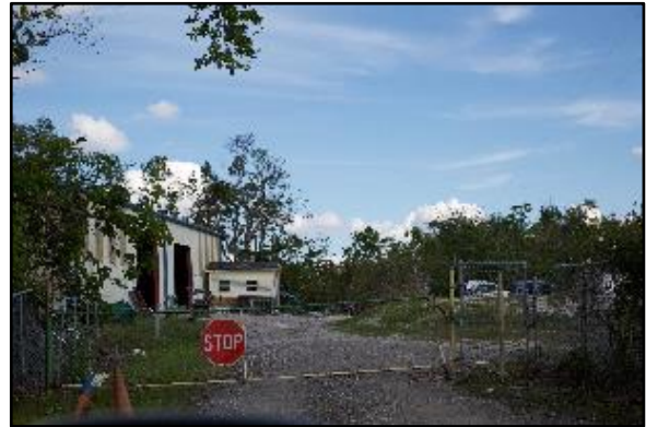
Figure 24: Everglades City Waste Water Treatment Plant
