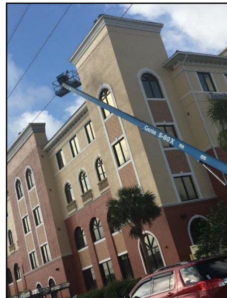
Figure 10: Repair of a Hospital - Cape Coral
